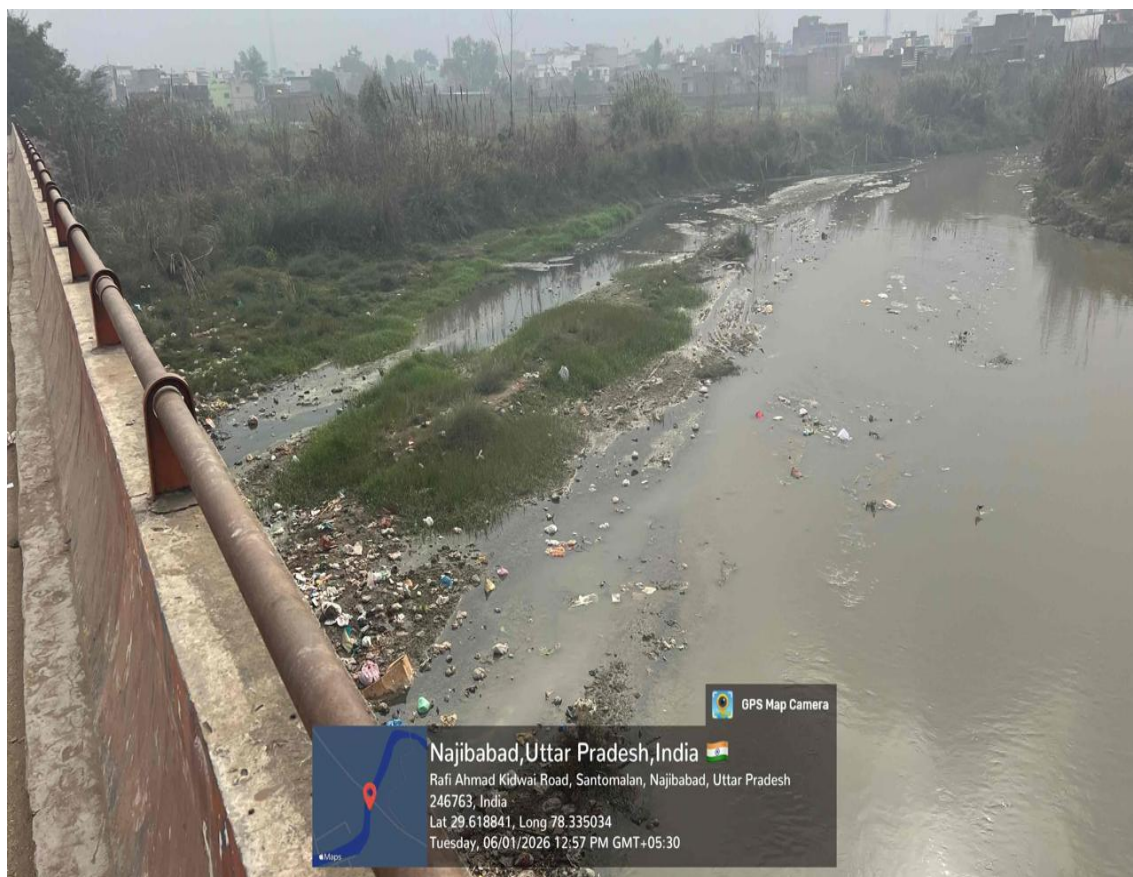
Figure 1: Encroachment in Malan River at Abufazar Colony
